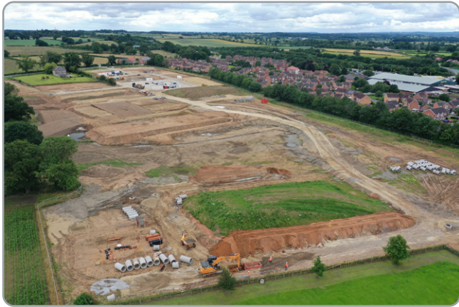
Sewer installation taking place on site
