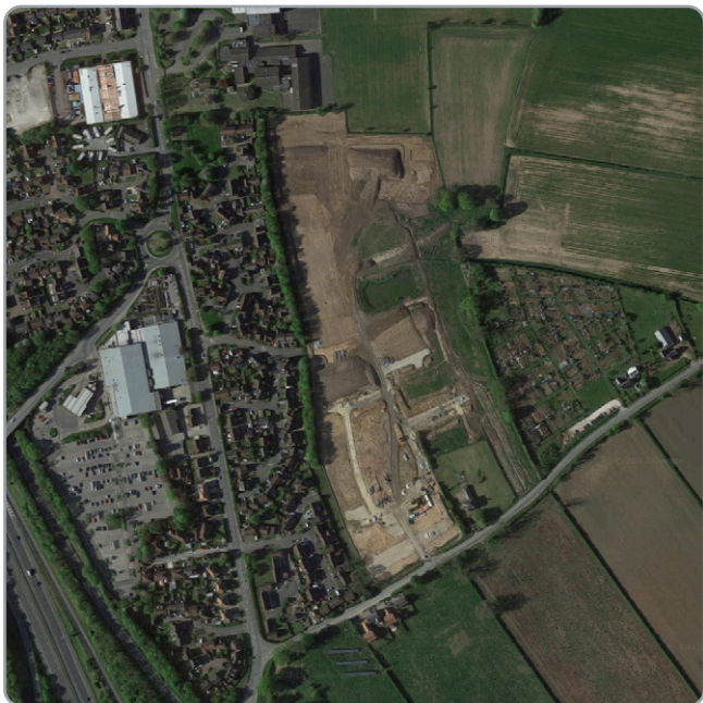
Aerial view of the whole site during initial phases
