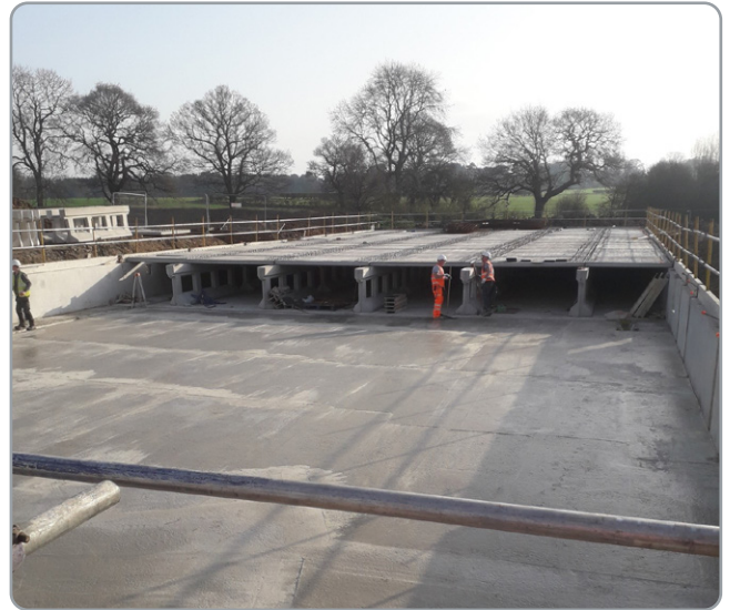
Installation of 1,051m 3 pre-cast concrete attenuation tank
