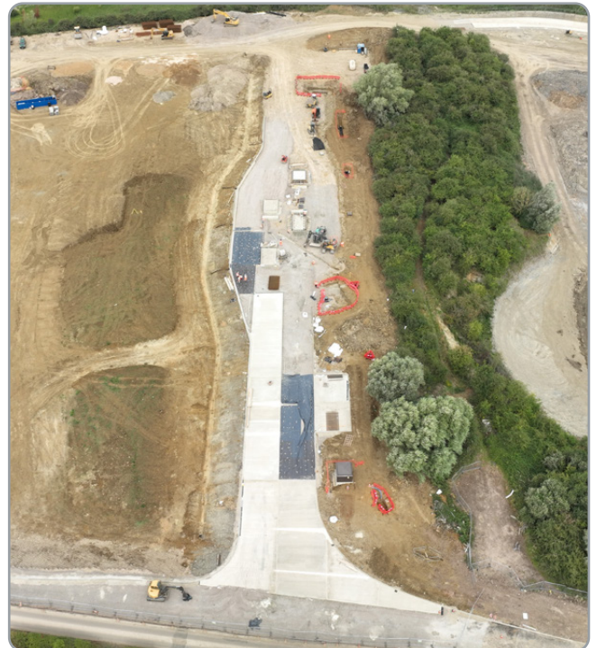
Concrete road way under construction
