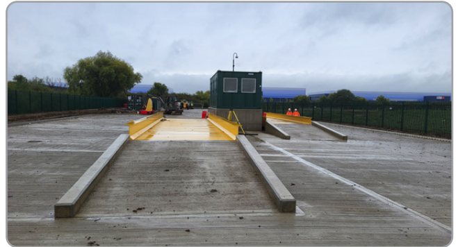
Nearing completion of construction works new weighbridge and offices installed
