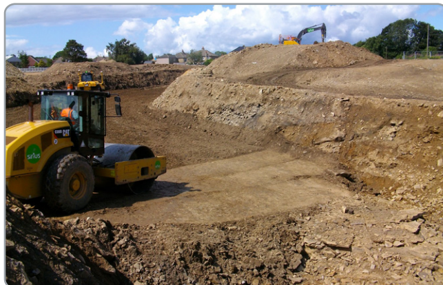
Compaction works
