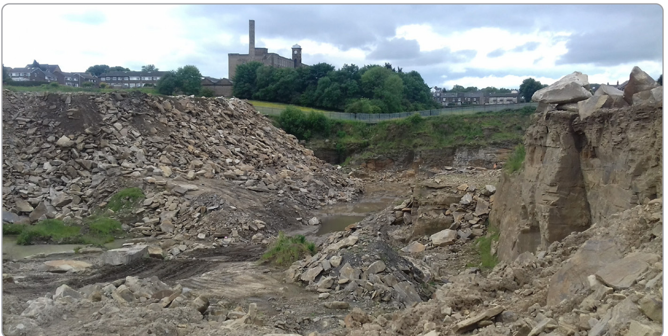
The former Fagley Quarry before commencement of Sirius works
