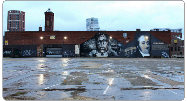
The old building at Southbank, Leeds before Sirius demolition works
