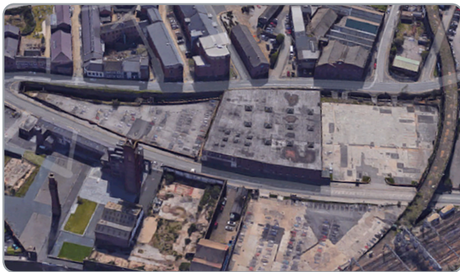
Aerial view of the site before demolition works started
