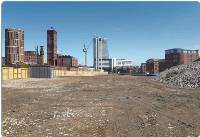
With Sirius works complete – the site ready for handover
