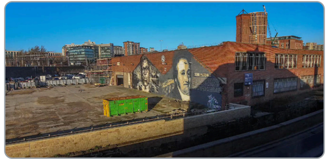
Site ready for the demolition phase
