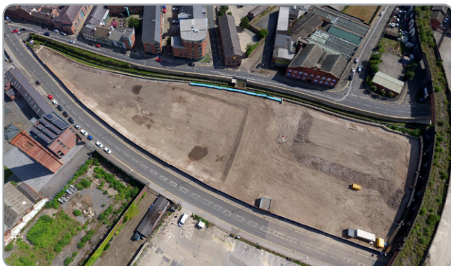
Final site view with Sirius works complete and ready to handover
