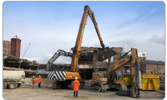
Building demolition well underway
