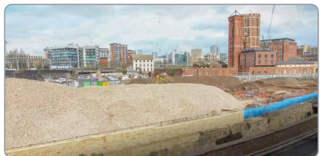
Creation of 6F2 stockpile from demolished/crushed material on site
