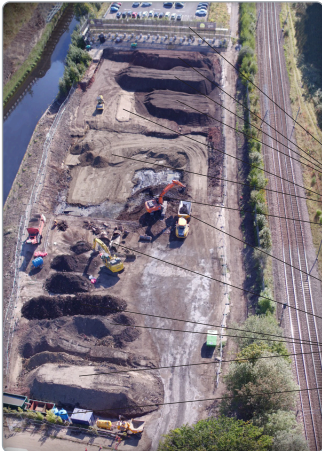
Kirkstall Forge – Plot K, excavation area
