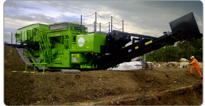
The Sirius STAR (Soil Treatment And Remediation) machine in action
