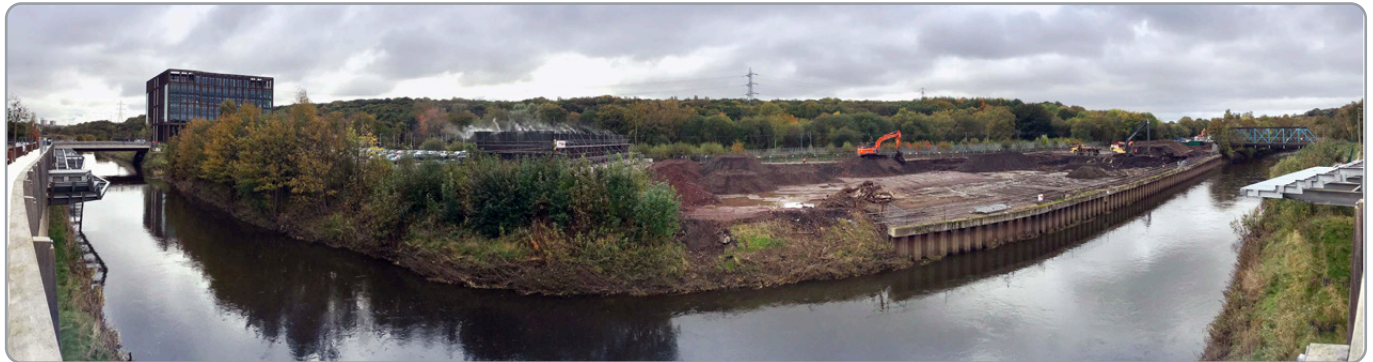
Excavations and remediation progressing well at the Kirkstall Forge site
