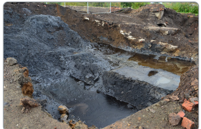
Contaminated soils being excavated in readiness for treatment
