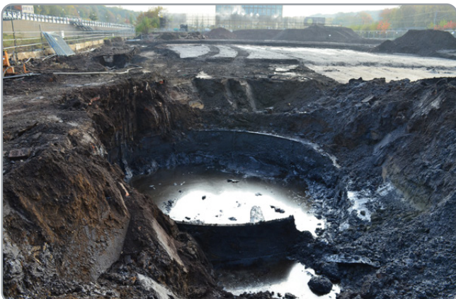
Excavations revealing the sites previous industrial use that had polluted many of the soils on site
