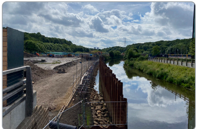
Ongoing construction of reinforced soil & Allan block wall
