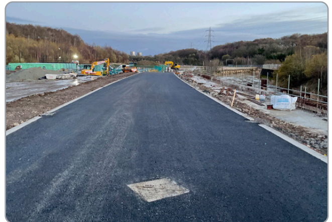
Construction of the river road
