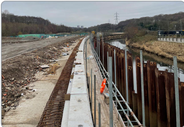
Ongoing construction of anchor slab and edge beam
