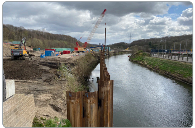
Installation of temporary sheet pile wall in the river
