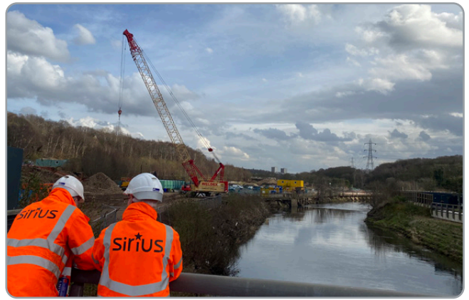
The crane arrives on-site ready to install the sheet pile wall
