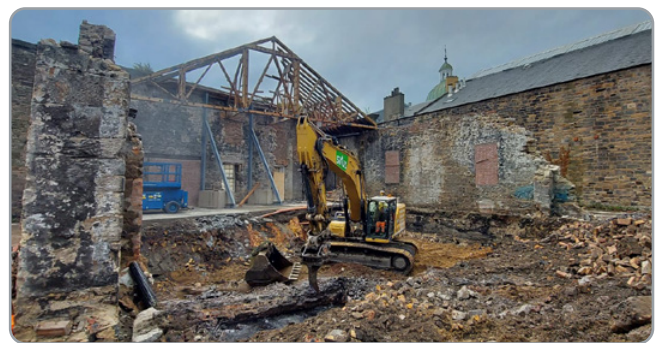
Final stages of the main former gasometer building demolition
