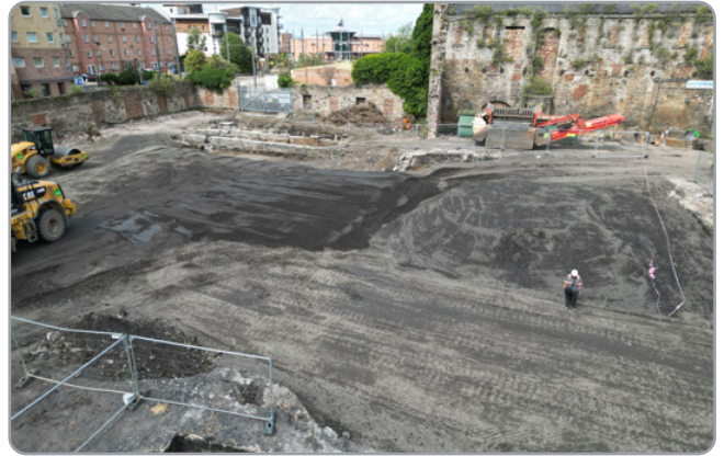
Reengineering treated materials within the former scrapyard
