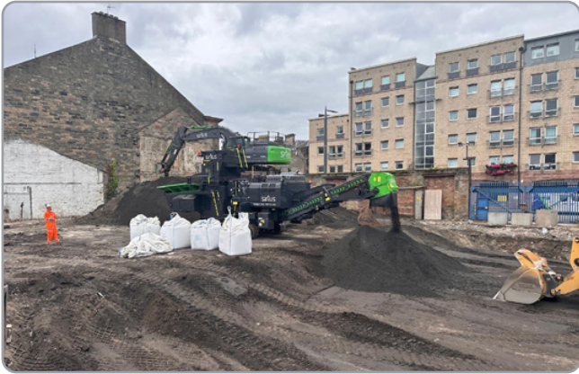
Treating contaminated soils using the MSR (Mobile Soil Recycler)
