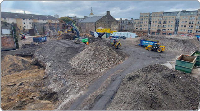
The site midway through the works
