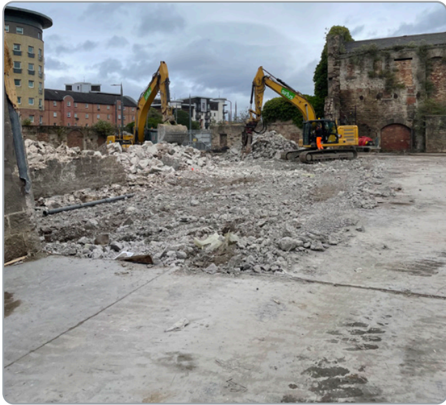
Breaking up the concrete hard standing within the former scrapyard
