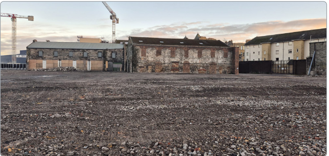
Sirius Enabling works complete
