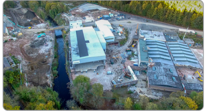
Sirius demolition phase of the former paper mill
