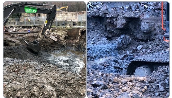
Contaminated soils being excavated in readiness for treatment
