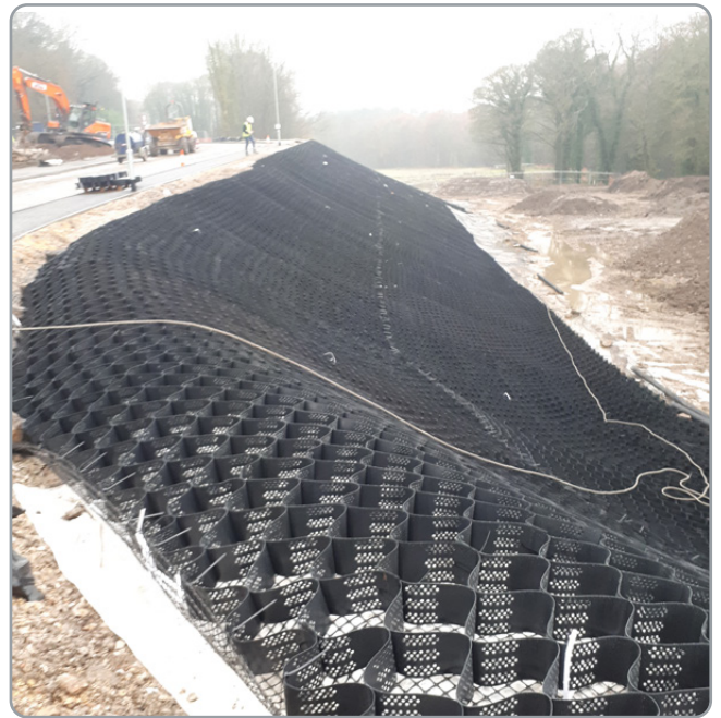
Highway embankment construction
