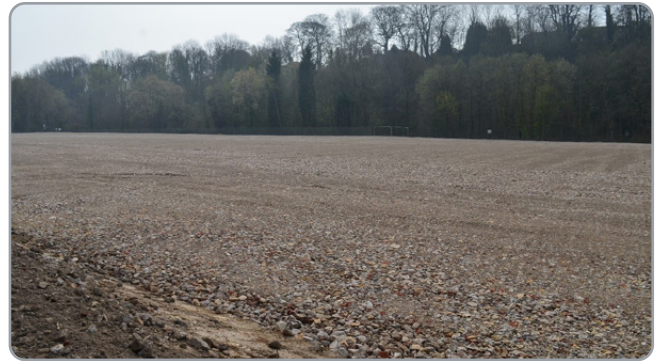
Final site surface ready for handover
