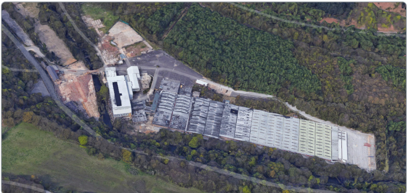
Aerial view of the former Oughtibridge Paper Mill
