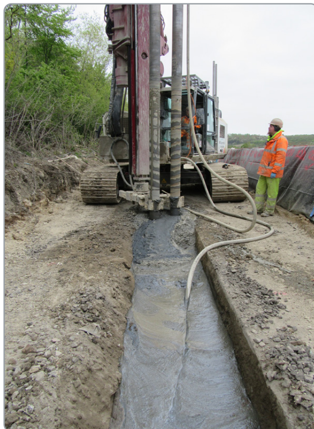
Grout and soil mix within leader trench
