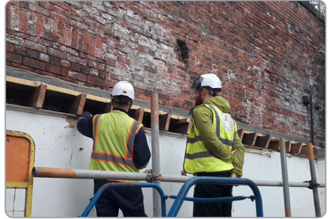
Careful inspection to make sure each stage is safe to proceed
