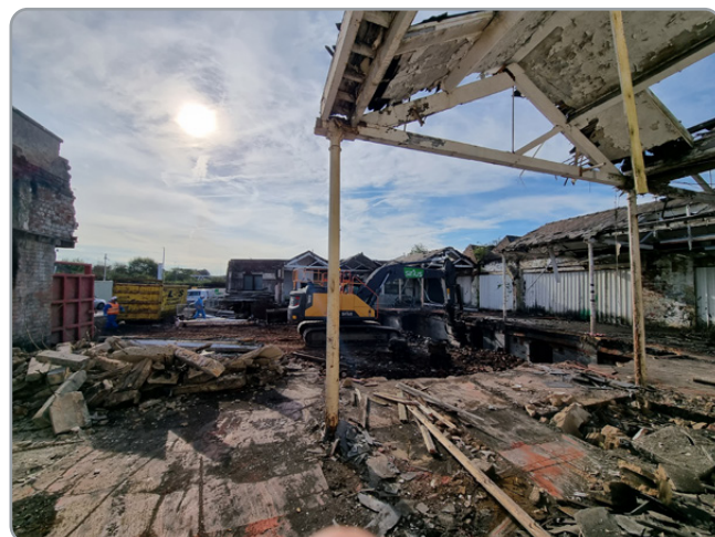
Demolition progressing in Building 3
