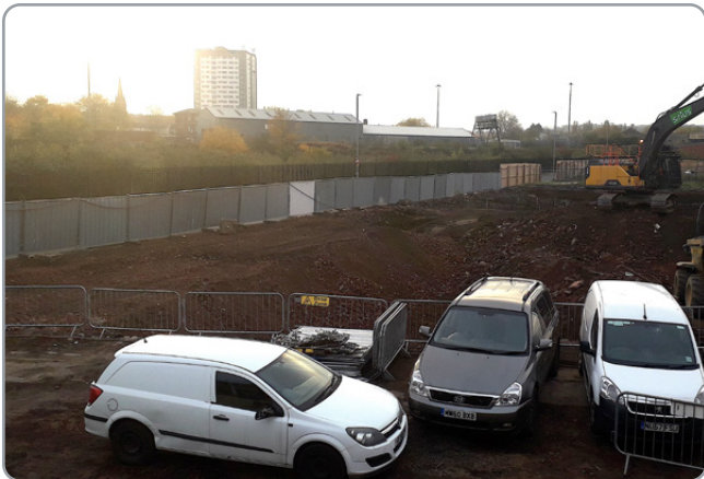
Sweet Street façade removed and replaced with temporary fencing
