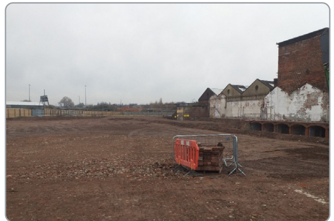
Completed site ready for development
