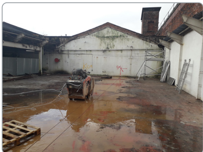
Building 3 Suspended floor - Saw cut along 5.0m off-set with Temple Works
