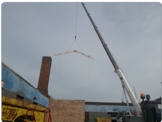
Steel roof trusses being removed by crane from Building 3
