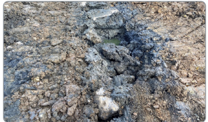
Hydrocarbon staining identified within opencast backfill
