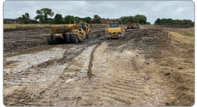
Topsoil strip within area KO1 undertaken by the Sirius Scrapper Team
