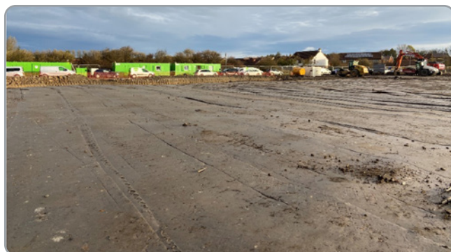
Finished remediated formation of BO3 looking north
