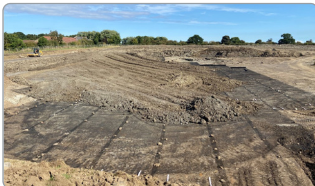
Placement of initial layer of engineered fill over geogrid within KO1
