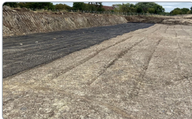
Placement of geogrid with minimum 0.3m overlap, at base of excavation
