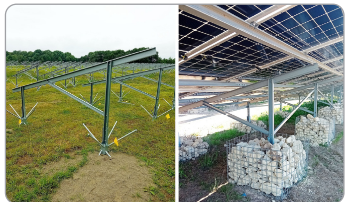
Alternative foundation types for solar panel frames
