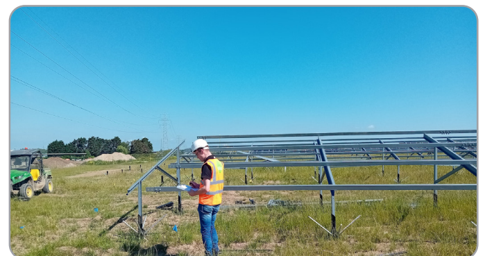
Sirius Quality Assurance Engineer checking construction
